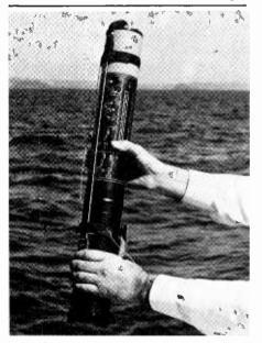
This floating beacon manufactured by Burndept, which has already captured orders worth £50,000 from Norway, operates on a primary battery and transmits on both the civil and military aviation distress frequencies (121.5 and 243MHz) for a minimum of 48hrs at 0°C. It measures 670  $\times$  85mm and weighs 2.89kg.
